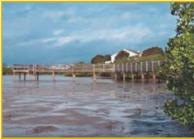
Ensuring vital habitats are protected when docks are constructed
