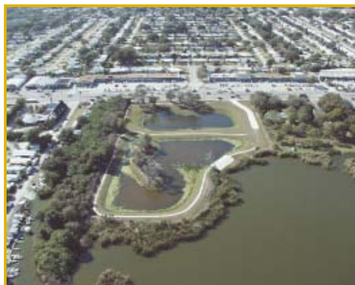
Lake Seminole stormwater treatment pond
