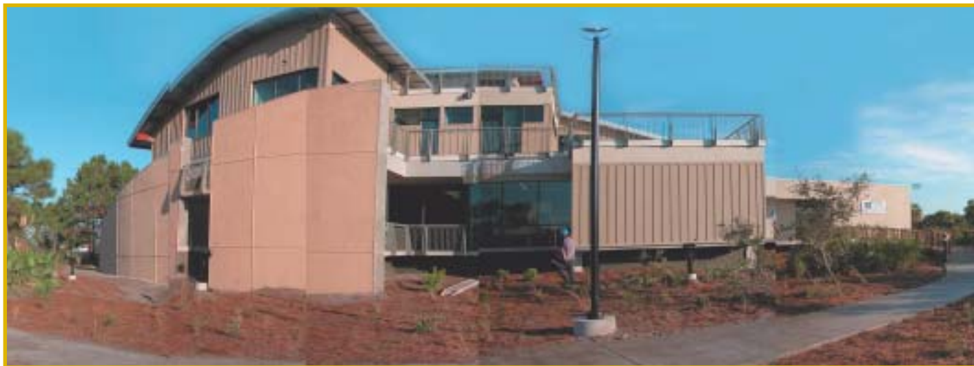
The Weedon Island Preserve Cultural and Natural History Center nearing completion
