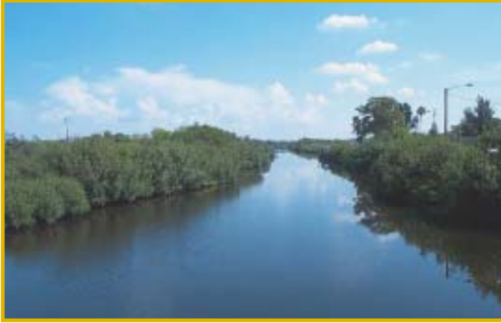
Cross Bayou Canal
